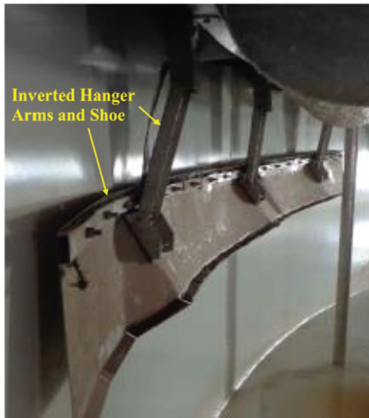
Figure 4. Overextension of mechanical shoe pivot linkage results in primary seal inversion.
